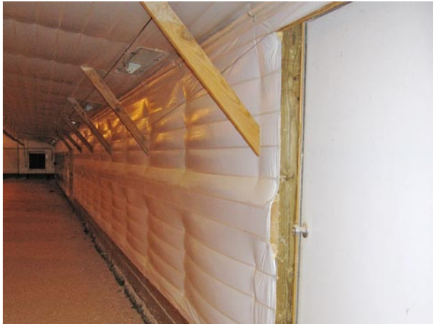
In wood-framed houses with posts on 4 or 5 foot centers, a low-cost insulation option is to fill the wall cavities with fiberglass batts and cover the interior with tri-ply with bands on 1-foot centers.
