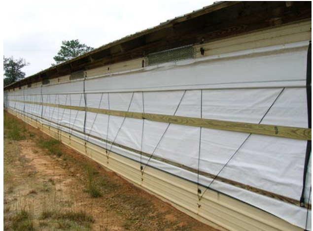
In low-cost energy retrofitting of a curtain sided house, the exterior curtains can be pulled good and tight and fastened with 1 x 4's, letting the existing curtain be the weather barrier. Exterior tin can be added later if desired.
