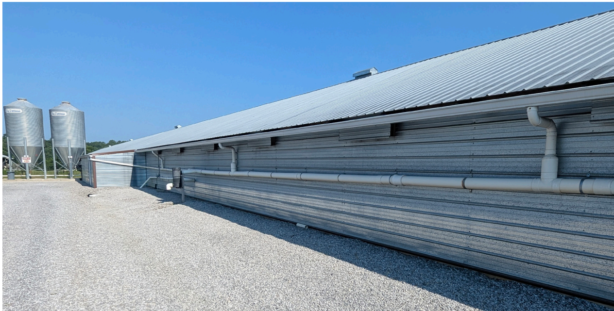
Figure 2. Rainwater is collected with gutters that feed through downspouts into collection piping. The black cylinder is a centrifugal prefilter that removes large debris before sending the water into underground piping to a storage bladder.
