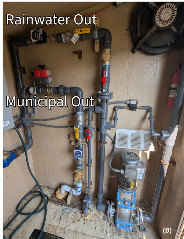
Figure 3. Inside the system control room (A), water is filtered through a bag filter to remove small particles before being disinfected through two ultraviolet (UV) lights. Control valves (B) are used to select between stored rainwater, when available, and municipal water for the four broiler houses.
