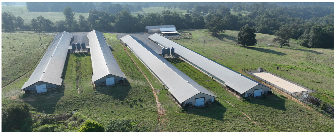
Figure 1. Aerial view of a four-house commercial broiler farm on terrain that slopes from highest to lowest points. The storage bladder is on the lowest terrain.
