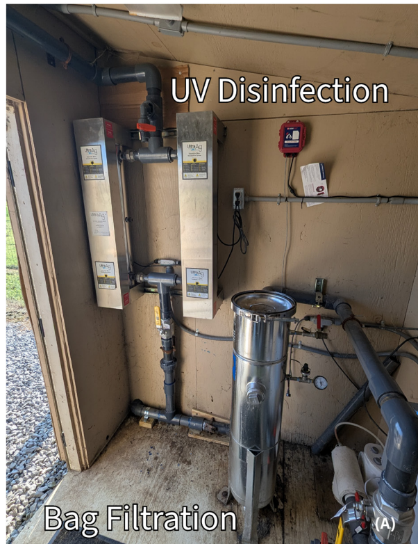
Figure 3. Inside the system control room (A), water is filtered through a bag filter to remove small particles before being disinfected through two ultraviolet (UV) lights. Control valves (B) are used to select between stored rainwater, when available, and municipal water for the four broiler houses.
