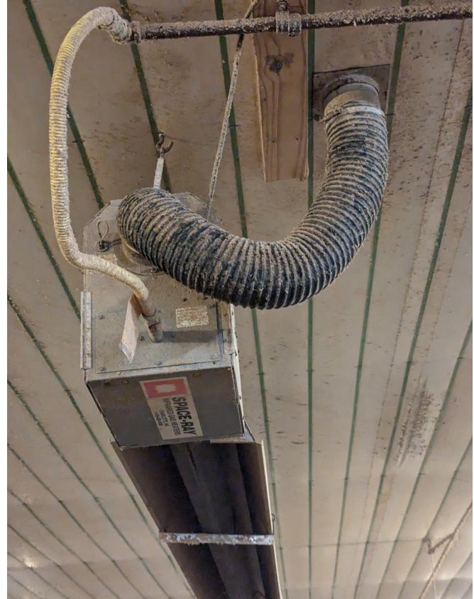
Figure 5. The air intake duct on this heater demonstrates how the duct length should allow a slight sag to trap condensation in the duct, reducing the moisture entering the heater burner box.
