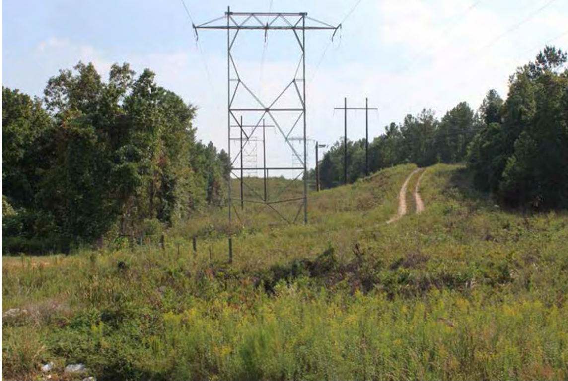
Figure 8. Ground view of utility swath/corridor (#3) in Figure 5
