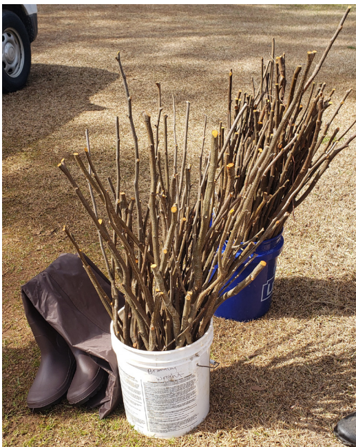
Figure 4. Cut live stakes stored for installation in a water bucket.
