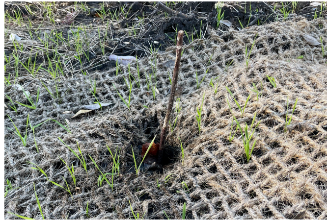
Figure 11. Live stake installed under erosion control matting at a stream restoration site.
