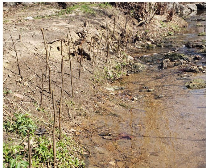
Figure 12. Live stakes installed along a stream.
