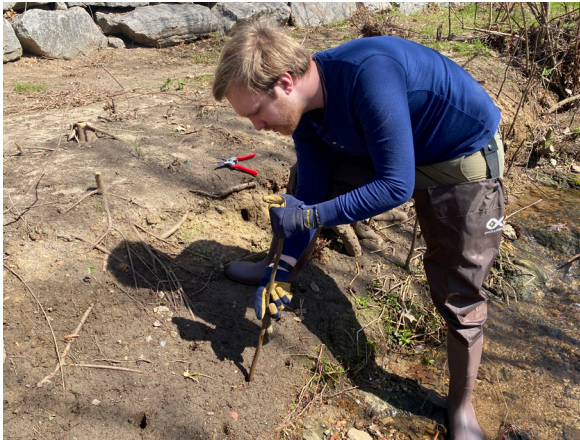
Figure 9. Installing live stakes next to a stream.
