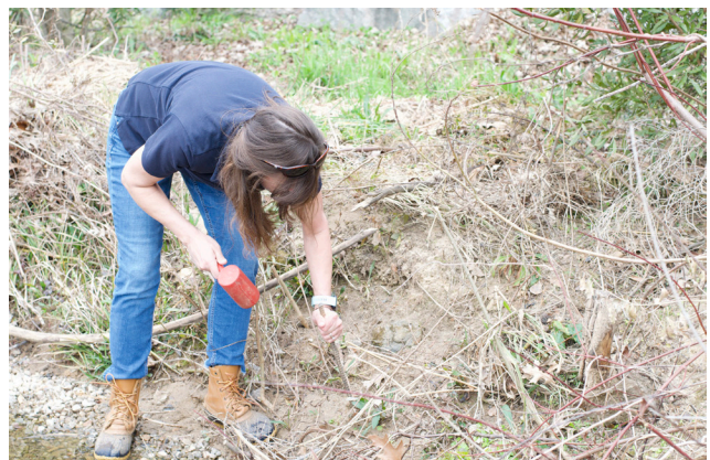
Figure 8. Use a piece of rebar or something similar to create a pilot hole. This will help prevent damage to the live stake.
