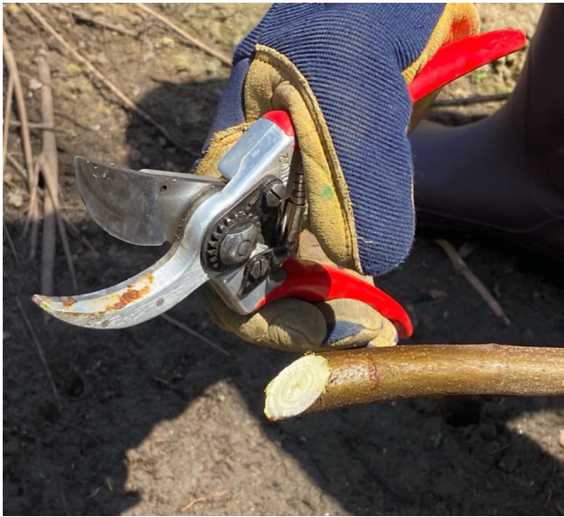
Figure 6. The end of a live stake is cut at an angle to make insertion into the ground easier and ensure that the stake is planted with the correct end facing up.
