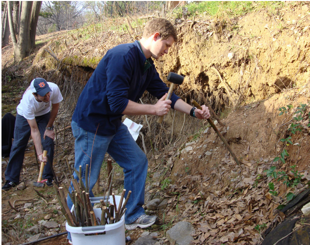
Figure 3. Live stakes being installed in an eroding stream bank.
