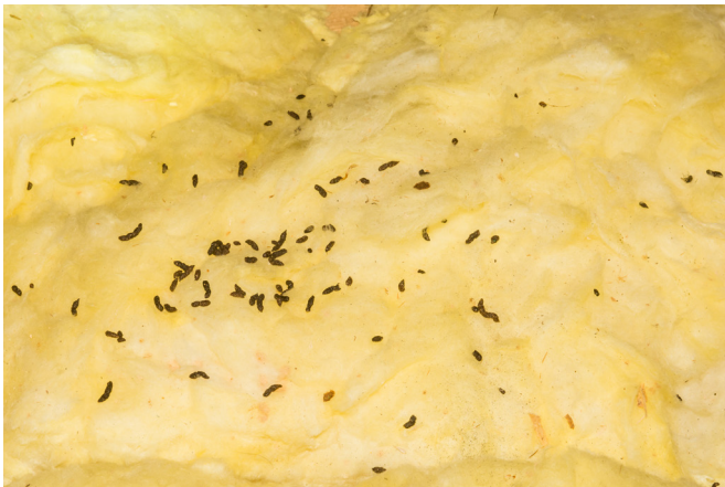
Figure 9. Bat feces on attic insulation.
