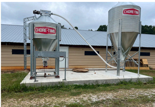
Figure 5. Each section or pen needs a small feed bin, scales, fill system, and hoppers.
