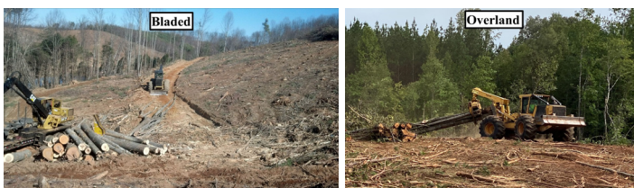
Figure 2. Bladed and overland skid trails.
