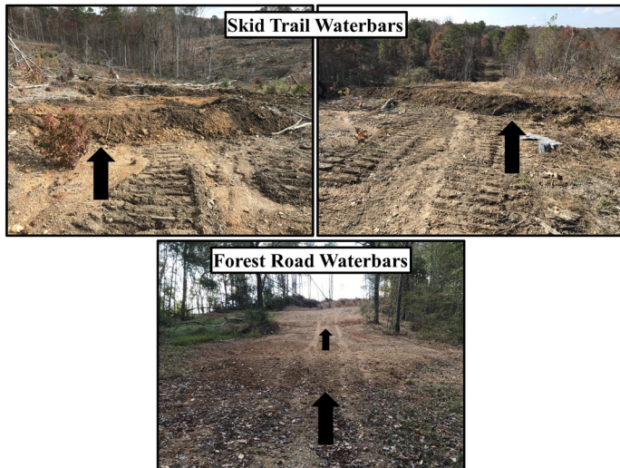
Figure 10. Skid trail water bars (top) need to be installed on sloped sections of skid trails. It is critical to install them on stream crossing approaches. Skid trail water bars can be larger and wider than forest road water bars (bottom) since they do not have to be designed for vehicle passage.
