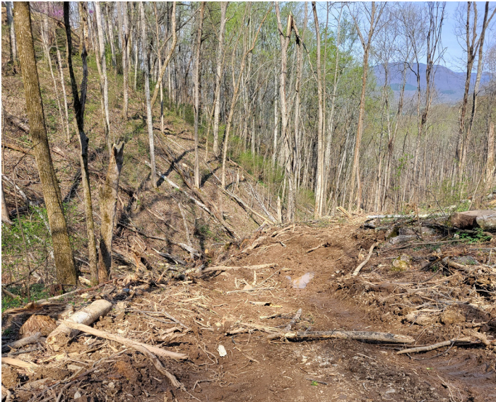
Figure 8. The skid trail was too close to the drain. Keep skid trails out of the streamside management zone (SMZ) except when crossing a stream. There also were no close-out BMPs implemented. (Photo credit: Andrew Vinson, Virginia Department of Forestry)
