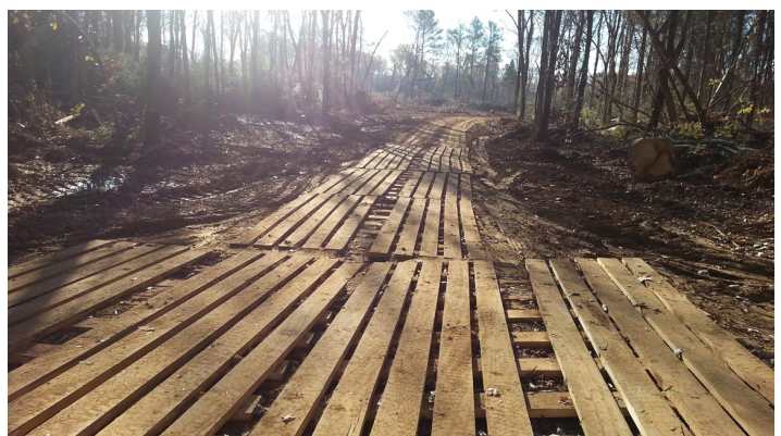
Figure 7. Wood mats work well to reduce soil rutting and compaction from forestry equipment.
