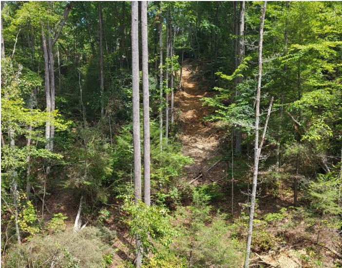
Figure 9. Steep skid trail that went directly into a drain and had no close-out BMPs implemented. (Photo credit: Andrew Vinson, Virginia Department of Forestry)
