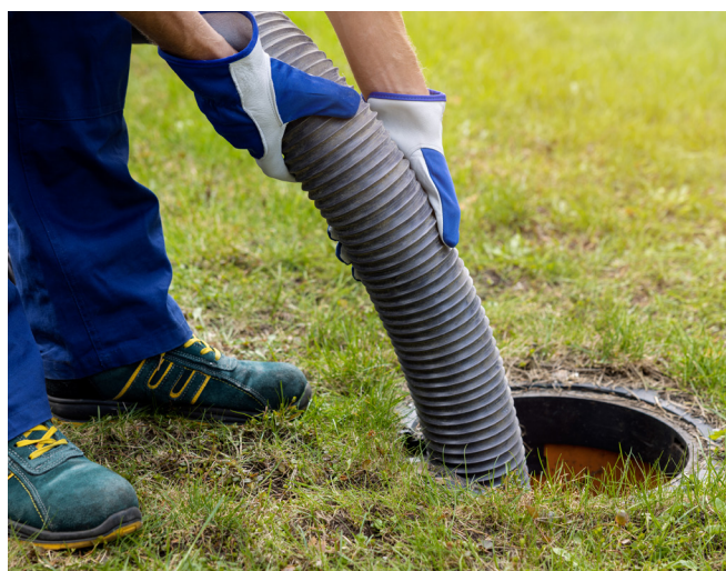
Figure 4. Inspect and pump out the septic tank.
