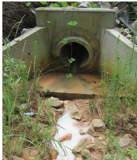
Figure 9. Paint discharging from outfall. (Photo credit: Dusty Kimbrow, Water Resource Management, Watershed Program Coordinator)
