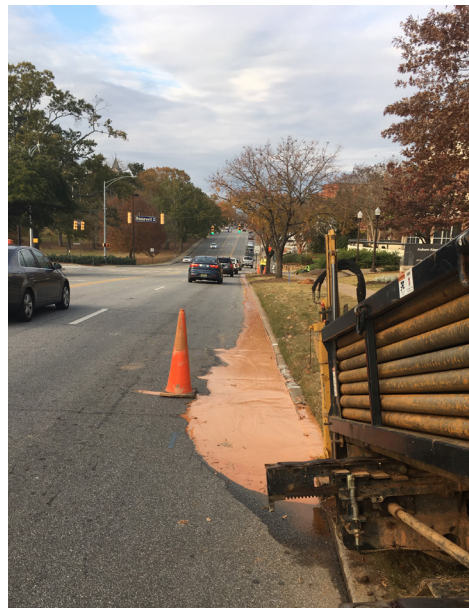
Figure 6. Mud entering a storm drain. (Photo credit: Dusty Kimbrow, Water Resource Management, Watershed Program Coordinator)
