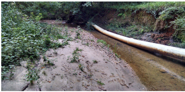
Figure 7. Exposed sewer line due to widening waterbody bank erosion. (Photo credit: Dusty Kimbrow, Water Resource Management, Watershed Program Coordinator)
