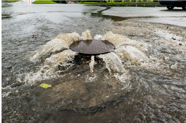
Figure 3. Overflowing sewer system. (Photo credit: Dusty Kimbrow, Water Resource Management, Watershed Program Coordinator)
