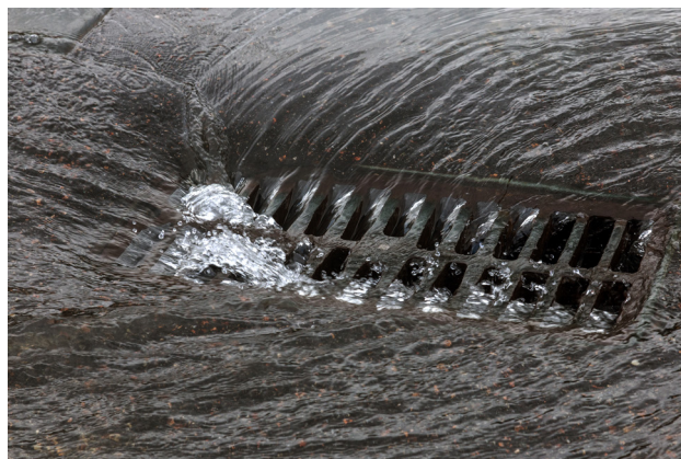
Figure 1. Storm drains can transport runoff known as nonpoint source pollution . (Photo credit: Dusty Kimbrow, Water Resource Management, Watershed Program Coordinator)
