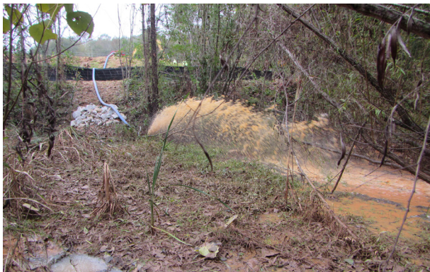
Figure 8. Water piped from construction site to creek. (Photo credit: Dusty Kimbrow, Water Resource Management, Watershed Program Coordinator)
