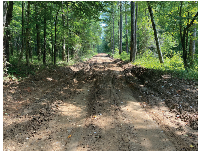
Figure 5. Critical road segment next to stream crossing (not shown) rutting and moving sediment toward a stream. Regrading and applying gravel are recommended.
