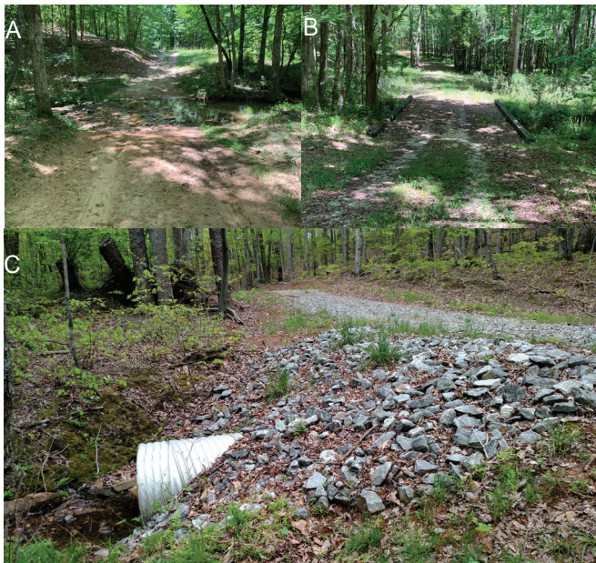
Figure 4. Stream crossing methods: (A) ford, (B) bridge, (C) and culvert.
