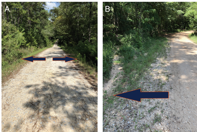
Figure 1. (A) Crowned forest road with ditches on both sides to get water off the road quickly and (B) ditch turnout to get runoff and erosion out of the forest ditch and into the forest.
