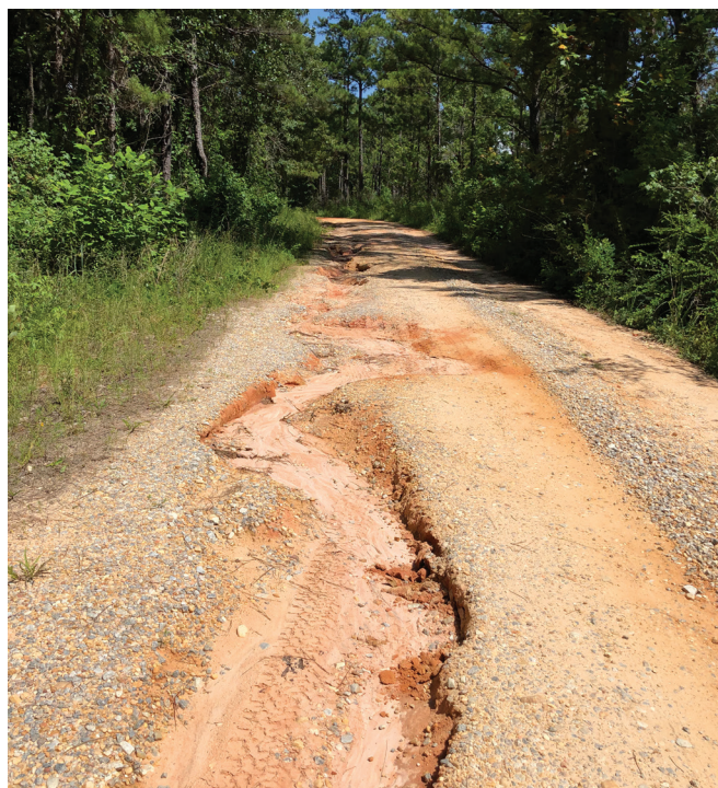
Figure 2. Forest road with erosion problems due to not directing runoff off the road.
