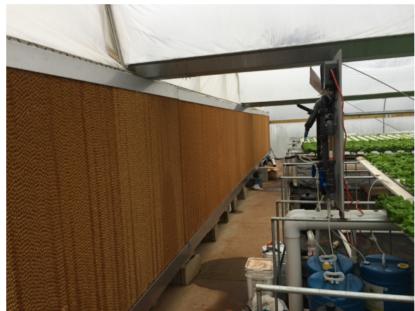
Figure 6. Evaporative cooling pad with cellulosic corrugated pad.
