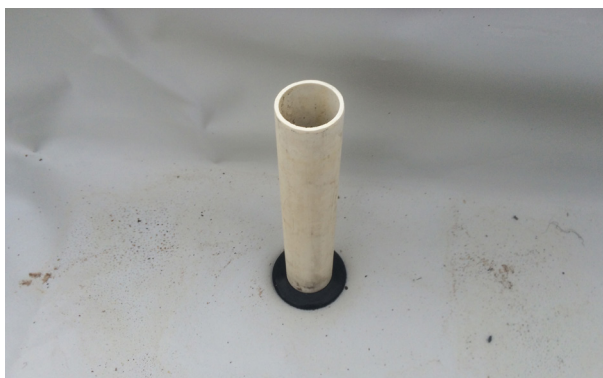
Figure 6. Standpipe in a DWC bed using a bulkhead fitting to plumb through the liner
