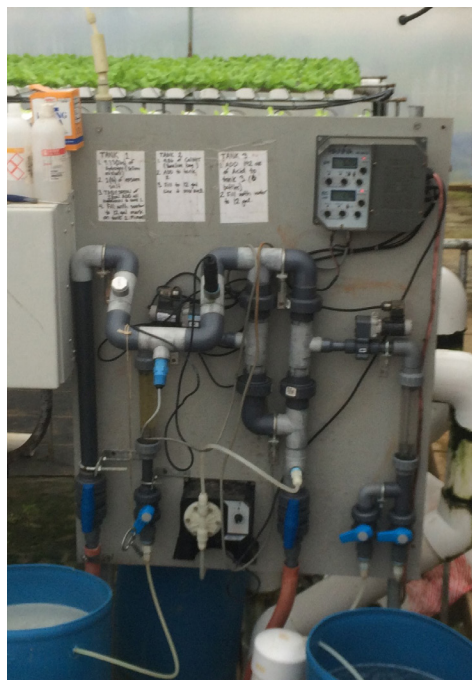
Figure 11. Computerized fertilizer dosing system.
