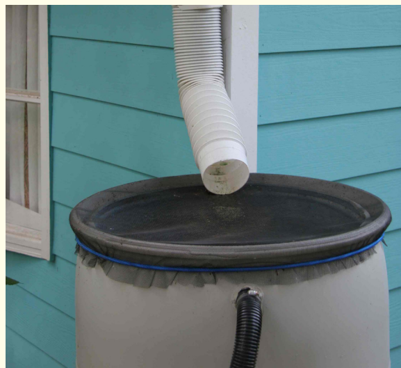
Rain Barrels are an excellent way of collecting an on-site resource and slowing the speed of water flowing off property.
