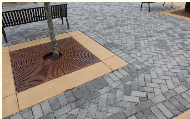
Permeable pavers are set in sand, gravel, a raised-grid structure, or a combination of these.
