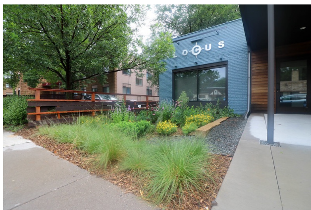
Figure 7. Rain garden installed in front yard to capture stormwater runoff. (Photo credit: Mississippi Watershed Management Organization, CC BY-NC 2.0)
