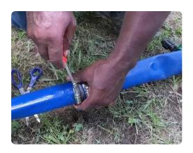
**Step 4.** Move the pipe clamps just past the barbs. Tighten them with a screwdriver.
