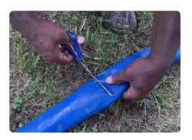
**Step 2.** Cut the lay flat in half right over the leak point.
