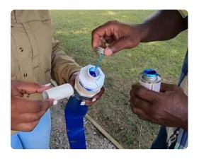
Step 5. Apply more PVC glue to attach a short 2- to 3-inch piece of PVC ¾-inch pipe.
