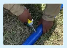
**Step 1.** Use a Phillips head screwdriver to punch a hole in the lay flat header. Leave the water on to make it easier to punch the hole. Use a screwdriver with a slightly smaller head than the fitting so it won't leak around the fitting.
