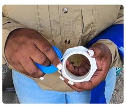
**Step 2.** Wrap Teflon tape around the threads on a 2-inch male PVC couplet. The tape must go on clockwise so it will not bunch up when you screw it into the gray barbed connector. Use pipe wrenches to make sure it is tight.
