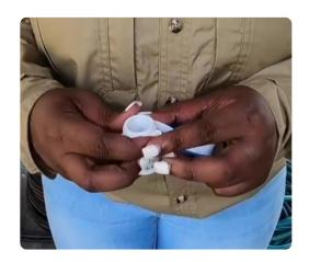
Step 4. Wrap the threads of a ¾-inch female connector with Teflon tape. Screw it into the reducer.
