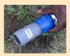
**Step 3.** Use a coupling or barbed splice fitting to join the two parts back together. Take two clamps and insert them on both sides of the pipe. Insert the barbed splice fitting into one side
