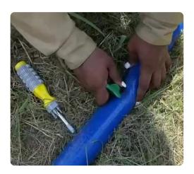
**Step 3.** Push the fitting into the hole. Listen and feel for a pop when the fitting slides in the hole.
