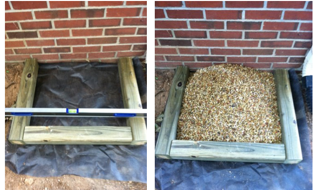
Figure 24. Make sure your platform is level before installing the rain barrel. Pea gravel can be used to create a supportive and easily leveled platform.
