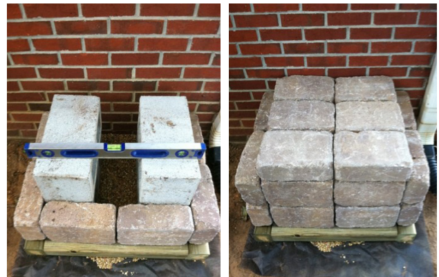
Figure 25. Make sure your rain barrel base is both level and secure. Elevating your barrel will increase your water pressure.
