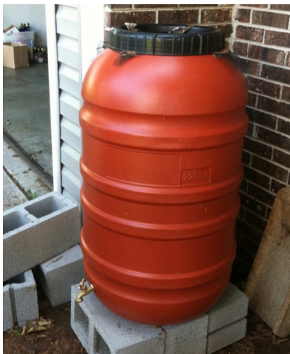
Figure 34. Finished rain barrel, slightly elevated, under gutter downspout
