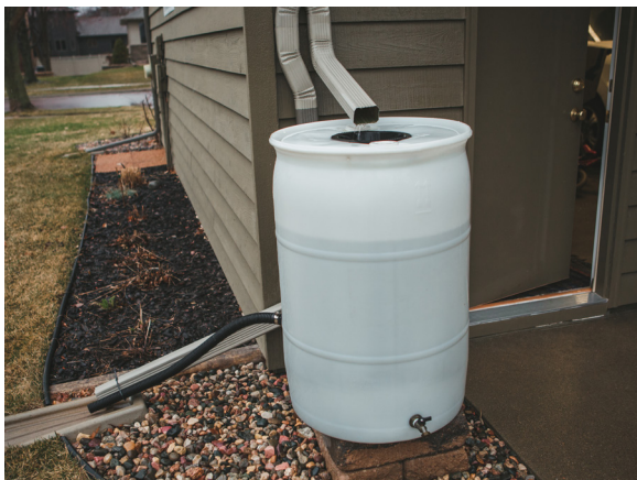
Figure 5. Catchment roof with gutters leads water into a conveyance PVC pipe, transporting water into a cistern.
