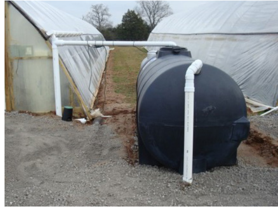
Figure 10. A 1,000-gallon rain tank, Moulton, Alabama
