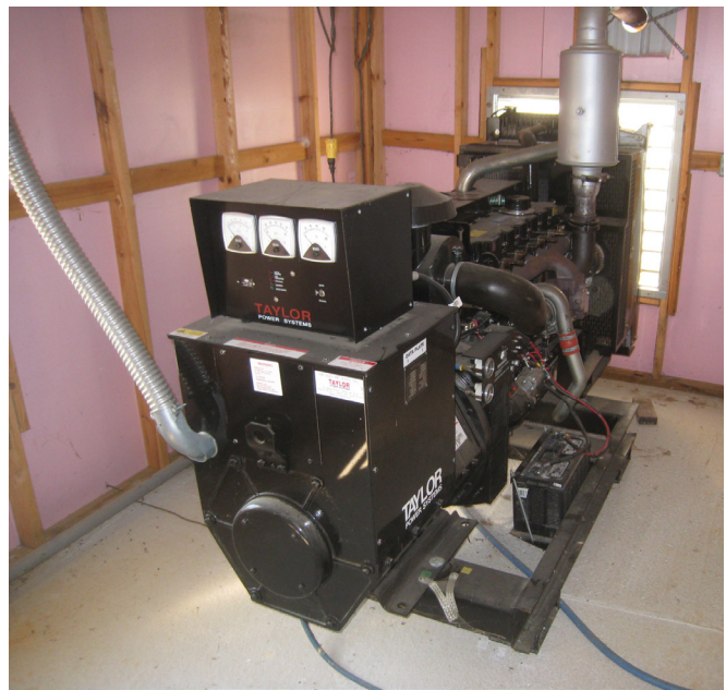
Figure 2. Typical poultry farm 100 to 175 hp backup generator.
