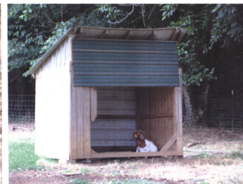
Figure 4. This structure is on skids and can be towed to another site using a tractor. (Photo by Sydne and Robert Spencer, Spencer's Farm)
