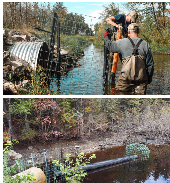
Figure 3. Excluding beaver access to culverts, drains, and spillways is a good damage-prevention practice. Installations can be simple, with metal posts and fencing used (top), or complex, with multiple fences and piping (bottom). Most any exclusion will require monitoring and maintenance to ensure they stay cleared. (Credit: USDA-APHIS Wildlife Services)
