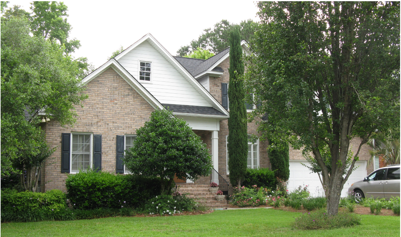
Several plants are too big for the area where planted.
