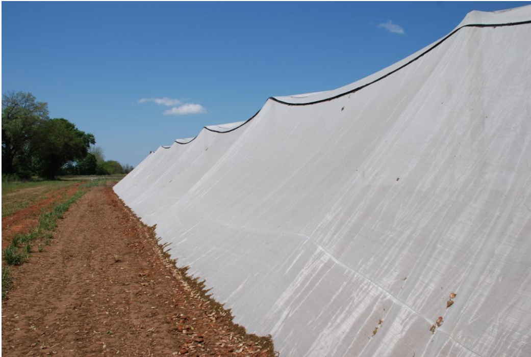
Fig. 2. The long side-walls of this net house are buried 2-3 feet into the ground providing strength and stability to the structure. The short side-walls were left open for planting operations.
