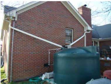
Storage tank and roof lines
