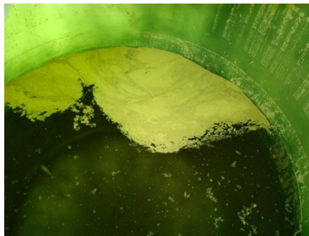
b. Tree pollen floating in an RCR tank after a storm event during
