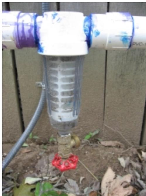
leaves and acorns from the water source prior to entering the first flush diverter. If your gutters are covered, a roof washer will probably be unnecessary. If you use trickle or drip irrigation, you should put in an inline filter after the pump (Figure 4). This will remove sediment that clogs trickle tubes and drip lines. The filter's screen size should be at least a 200 mesh. Remember, the larger the mesh size, the finer the screen.
