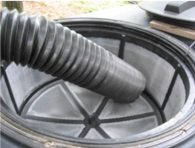
**Figure 5. A screened basket in the manway hole will prevent a lot of organic matter and mosquitoes from entering the tank.**
