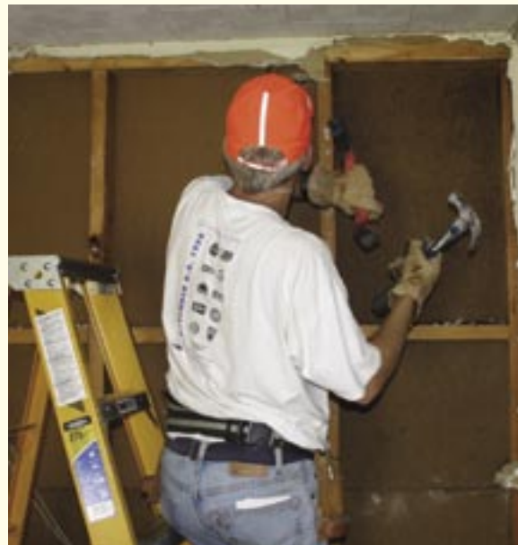
This volunteer tears out a wall to prepare for rebuilding.
