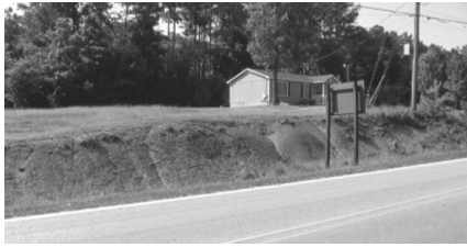
Figure 1. Eroded soil can wash down drains.
