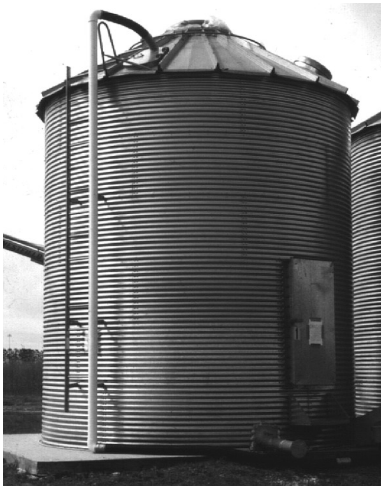
Figure 8. The gas is pumped up through the bin and then pulled down through a pipe running along the outside of the bin.
