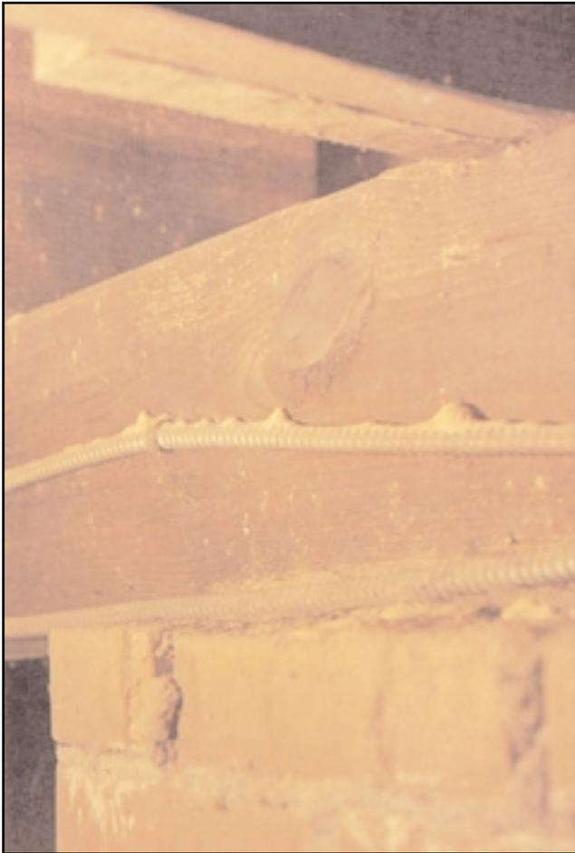
Powdery wood dust from powderpost beetles often collects in piles in crawl spaces.
