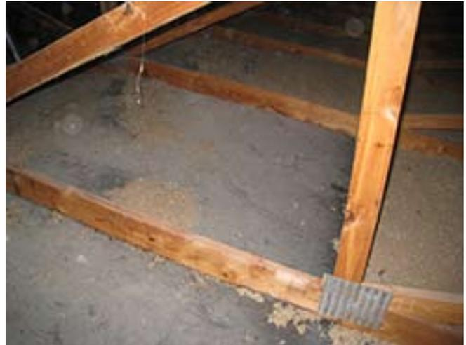
Photographs above were taken in north Alabama in a house about 10 years old. Notice the bare ceiling material in the middle of the house and the exposed lumber at the bottom of the trusses, showing that the blown-in insulation has not only shifted but thinned out. If your insulation looks like this a new insulation job should be at the very top of your list of things to do.
