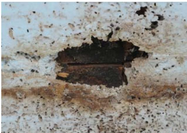
**Darkling beetles burrow into wood and foam insulation in search of food and for dark places to pupate. The damage to houses they cause can easily run to several hundred dollars per house per year. Photo shows damage to blueboard insulation. Damage like this – happening throughout the house, as it often does when beetles are not controlled – will seriously impair house heating and cooling efficiency. This means poor flock performance resulting from less than optimum in-house conditions.**
