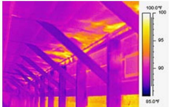
Above left thermal photo, taken during hot weather, shows temperatures in the 90s and above along the centerline where blown-in insulation has shifted, compared with temperatures in the 80s along the rest of the ceiling. Right photo shows hot spots in another house where insulation has been blown by wind away from the sidewall area. In both houses, additional ventilation will be required and it will be harder to maintain an optimum growing environment for the birds.
