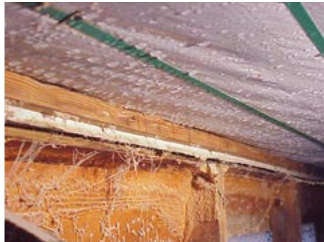
Condensation areas on ceilings such as this during cold weather is a good sign that insulation has been moved or is not in place in the attic. If left unattended, the constant accumulation and dripping of moisture will induce mold growth and cause damage to the house structure and any equipment that is continually kept wet.
