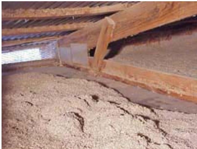
An inspection of insulation in the attic of this chicken house reveals that wind has most likely shifted insulation. Note the bare ceiling. When cold air in the attic comes in contact with the ceiling tri-ply in the attic, we will have condensation in the bird chamber as warm in-house air contacts the chilled tri-ply.
