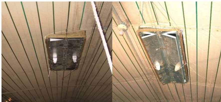
Figure 2. Attic inlets installed in ceiling of broiler house.
