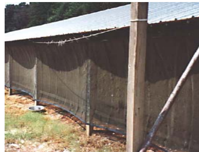
Shade cloth shields pads from sunlight.
