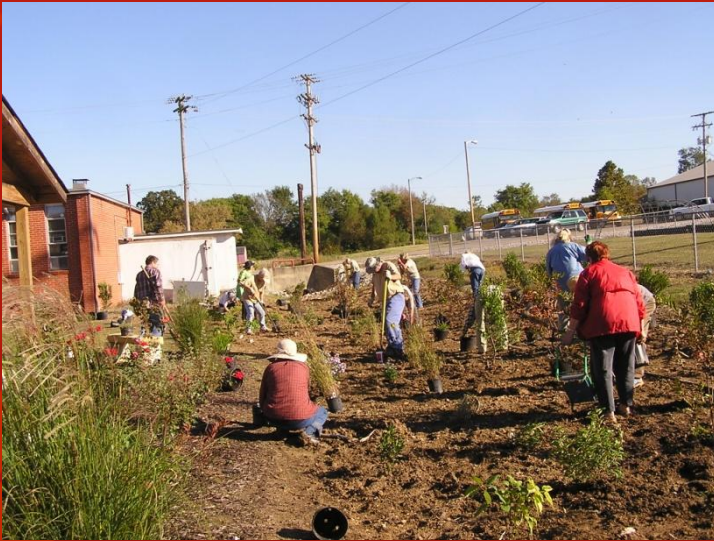
Shoals Area MG's install a rain garden at Anderson School.
