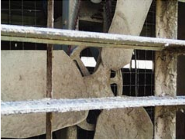
Photo at right is a close-up view of a fan blade that has not been cleaned for several weeks. The dust and dirt build-up changes the aerodynamics of the blade and puts additional drag on the blade, severely reducing fan performance.
