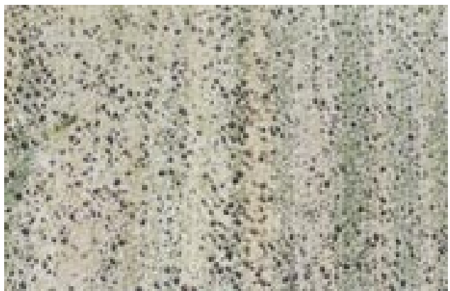
For most efficient and effective pad cooling, pads must be thoroughly wet. For recirculating pad systems, it is important to check headers regularly to be certain there are no plugged holes in the discharge pipe. Photo at left above shows properly functioning header. Right photo shows a thoroughly clogged pad. Flushing pads with water and using one of the widely available cleaning products helps prevent pad clogging. Clogged pads raise static pressure, reduce fan cfm's and wind speed, and reduce both real and wind-chill effective cooling.
