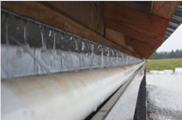
For most efficient and effective pad cooling, pads must be thoroughly wet. For recirculating pad systems, it is important to check headers regularly to be certain there are no plugged holes in the discharge pipe. Photo at left above shows properly functioning header. Right photo shows a thoroughly clogged pad. Flushing pads with water and using one of the widely available cleaning products helps prevent pad clogging. Clogged pads raise static pressure, reduce fan cfm's and wind speed, and reduce both real and wind-chill effective cooling.
