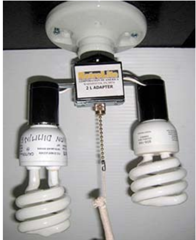
New dual bulb pull-chain adapters allow switching one bulb on or off at a time, as well as installing one dimmable and one non-dimmable bulb, as shown in photo above, without requiring additional wiring. Both bulbs are typically used during brooding; after turnout, when much lower light levels are required, the receptacle is switched to the dimmable bulb only.
