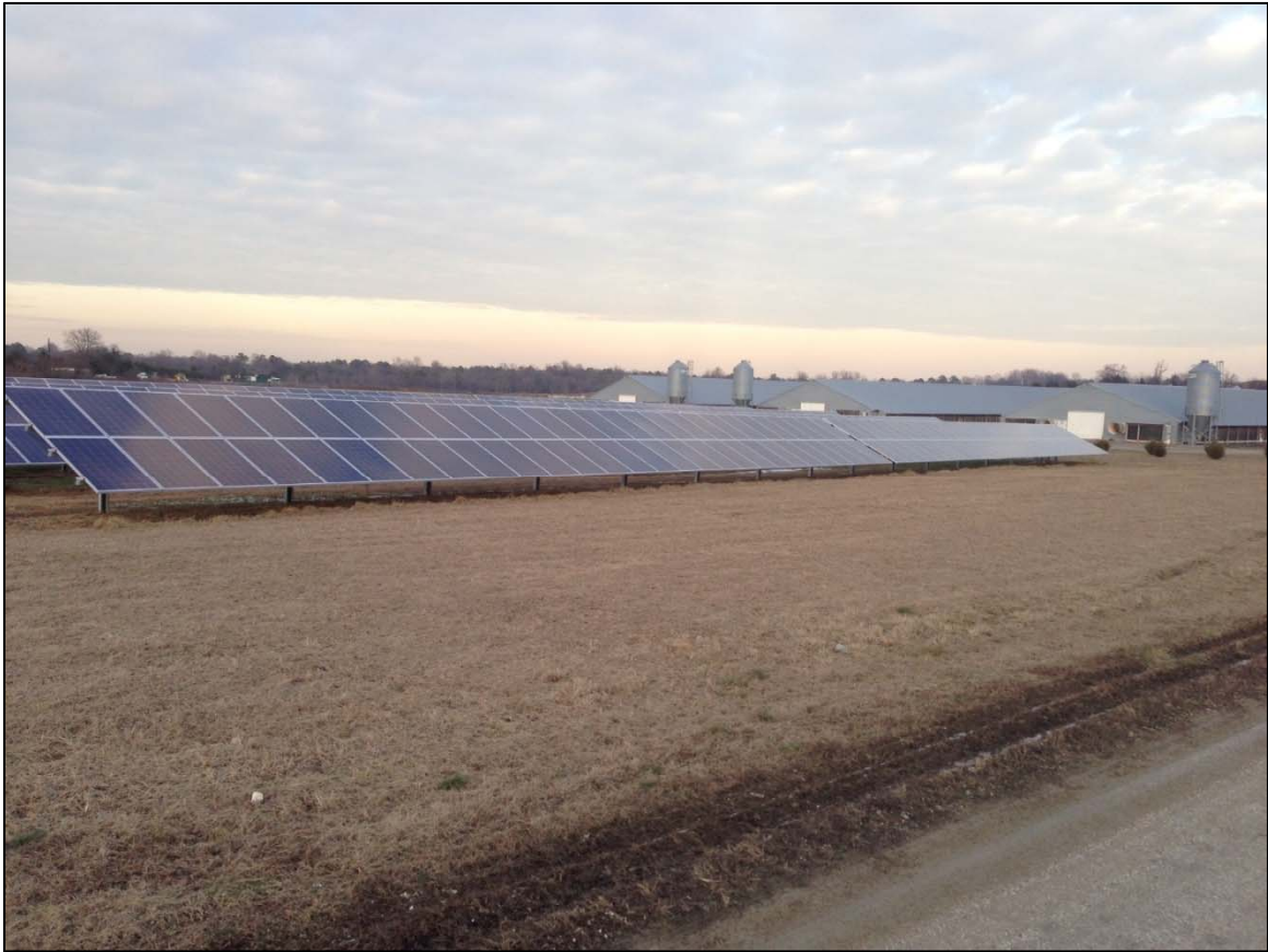
Figure 3: Ground mounting of the solar system is also a viable option. There can be many reasons to choose a ground mounted system, including aesthetics or houses not facing in an optimal direction. These systems work the same way and typically do not cost much, if any, more than a roof mounted system.
