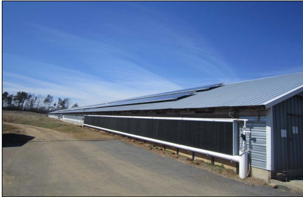
Figure 1: Solar panels take up little space on an average poultry house. Here we see a 100 KW system on a 40'x500' house. The size and weight of this system pose no threat to the stability of this house. The installation design also allows for modular replacement or repair of the panels if needed. Poultry houses with southerly facing roofs are ideal mounting places for solar systems.
