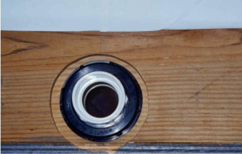
Picture 2 Illustration of the 2” bulkhead fitting set into the outside of the bed wall.
