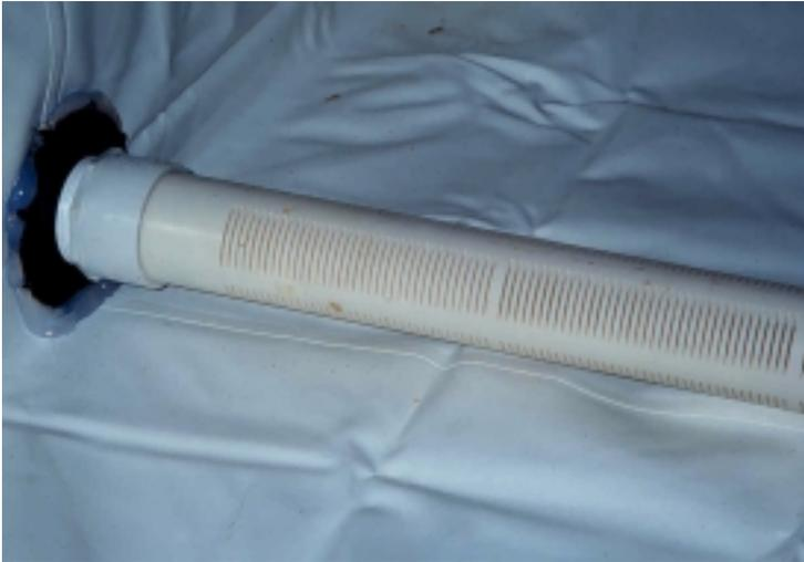
Picture 1 Illustration of the 20 mil plastic bed liner and bulk head fitting and well screen - drain.
