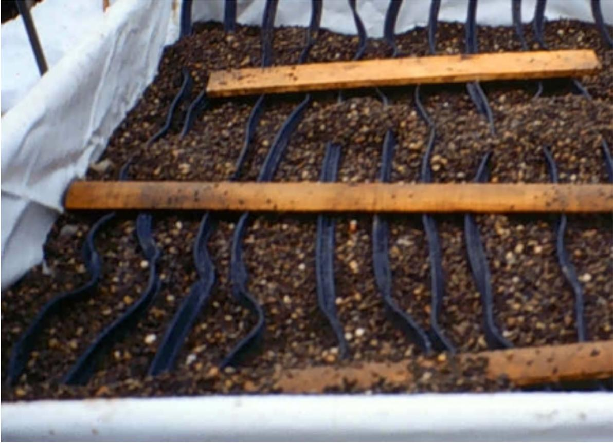
Picture 3 Illustration of the root-zone heating system buried in the gravel beds. Note boards were used to hold down the plastic tubing when filling the beds with gravel.
