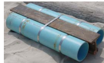
Figure 11: Example of pipeline weighted with railroad rail.
